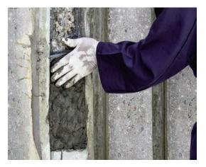
The product can be applied up to 15mm in thickness in vertical, unsupported situations and up to 40mm in recessed, supported repairs. The product can be applied in 100mm layers in the horizontal plane. The material should not be applied at less than 10mm thick.
